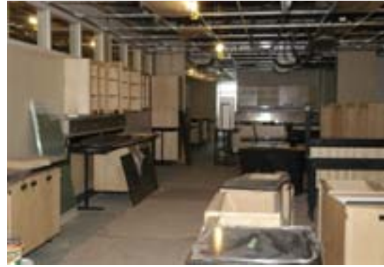
Another look into the new Chemistry Department.
