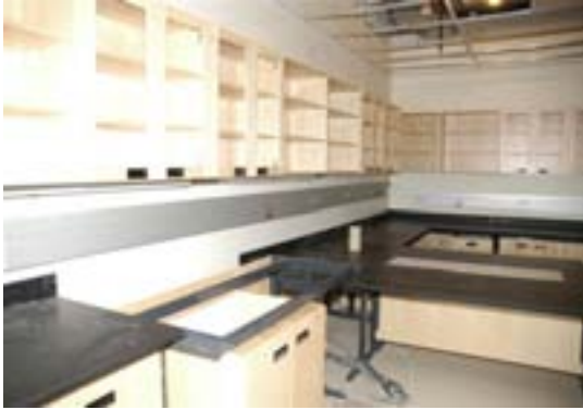
A view of the Microbiology area in the new building.
